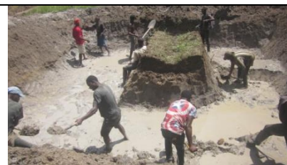
Construction of fish pond (10m x 10m ) in Maron Community
